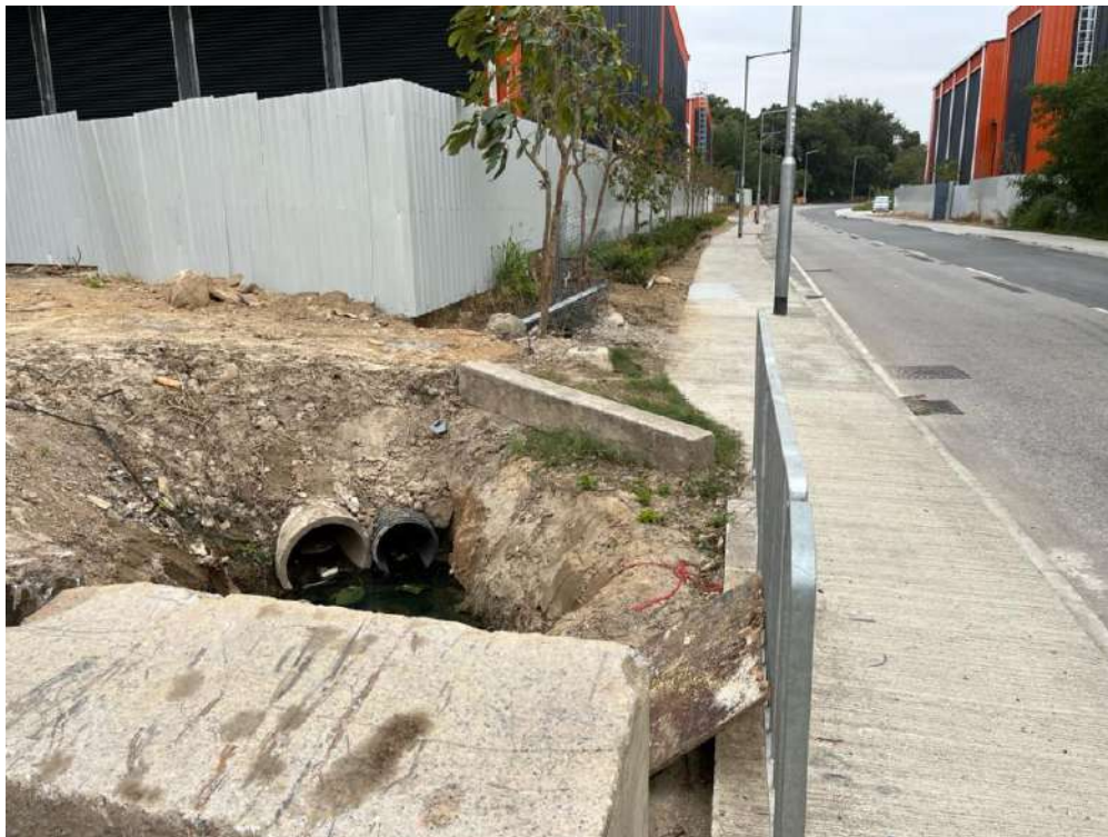
Plate 10 – Catchpit at Southern Side of Lin Ma Hang Road
