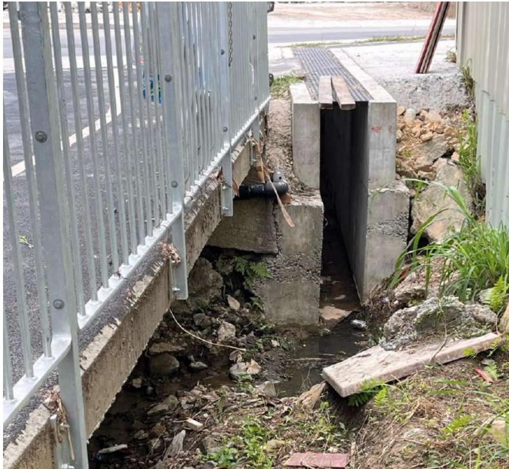
Plate 9 – Drainage Crossing Beneath Lin Ma Hang Road (view from the North)
