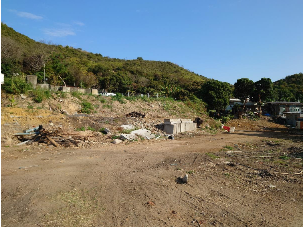
General view at southeast portion of man-made cut slope
