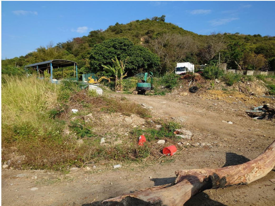
General view at south portion of man-made cut slope
