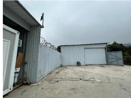
Existing Structure in the Application Site
