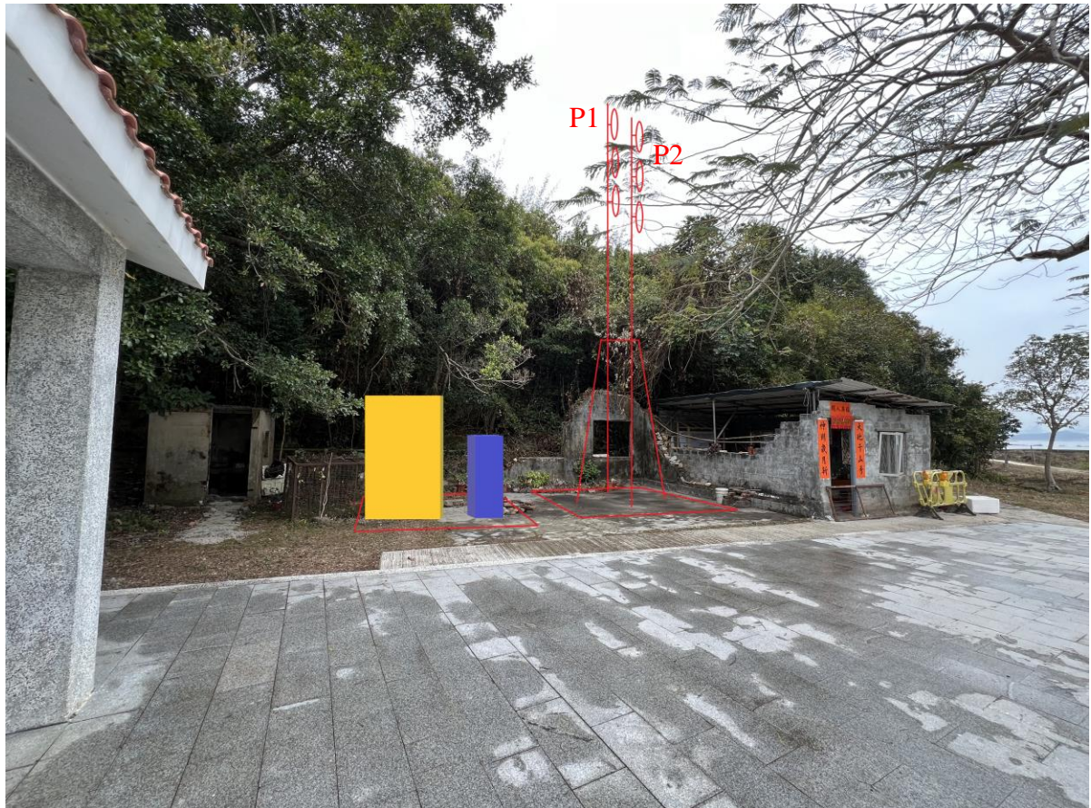
Photo 1: Showing the proposed antenna & equipment concrete footing location
