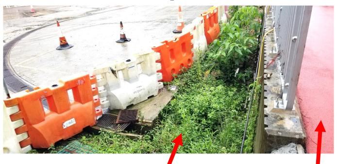
Space reserved for public drainage system. The existing 300mm UC will connected to the public drainage system which will be constructed by HyD.
