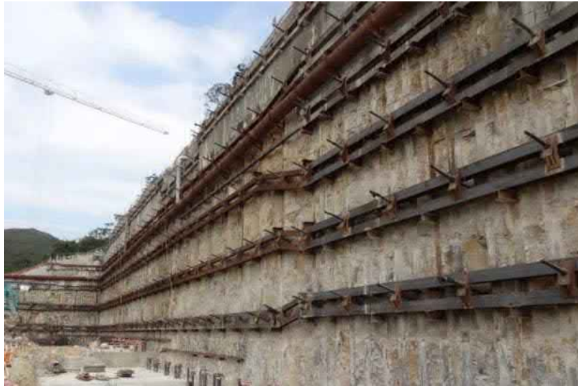
Reference Photo of Tieback System
