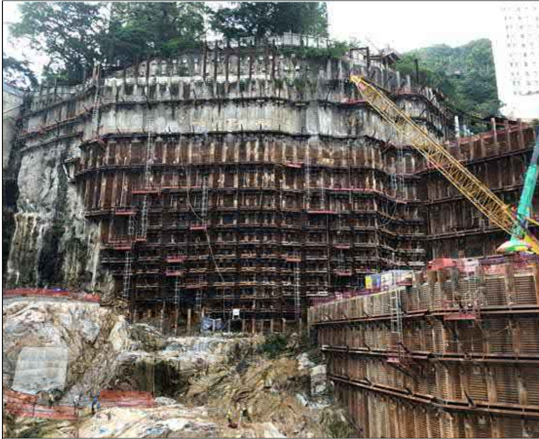
Photo 3: Temporary Tie-back of Hopewell Centre II
