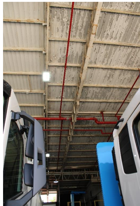
Photos 3.1 (Left) and 3.2 (Right): The Existing Fire Extinguishers and Automatic Sprinkler System
