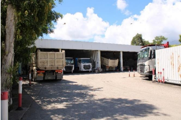
Entrance of the Site
