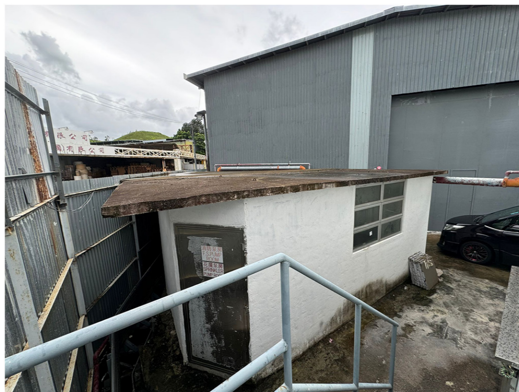
Fire Service Pump Room and Sprinkler Pump Room
