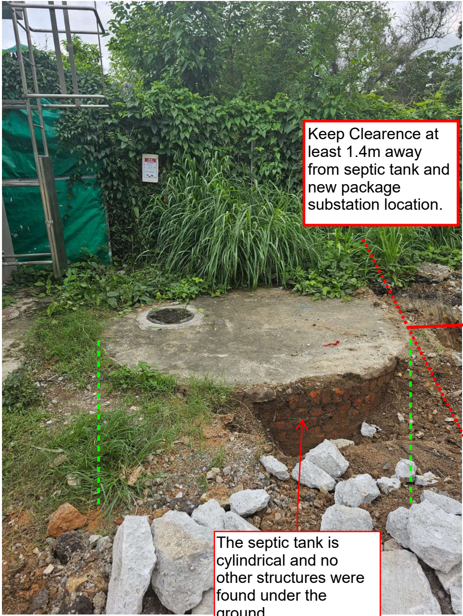
~ Trial hole for septic tank
