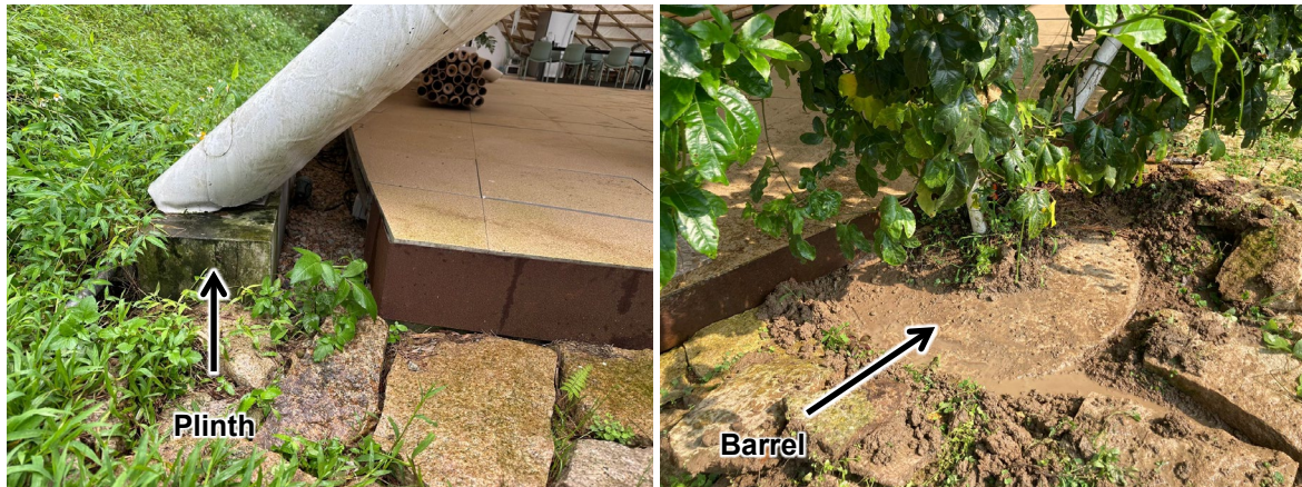
Figure 4.4 The Plinthes and Barrels of the Standalone Bamboo Shelter
