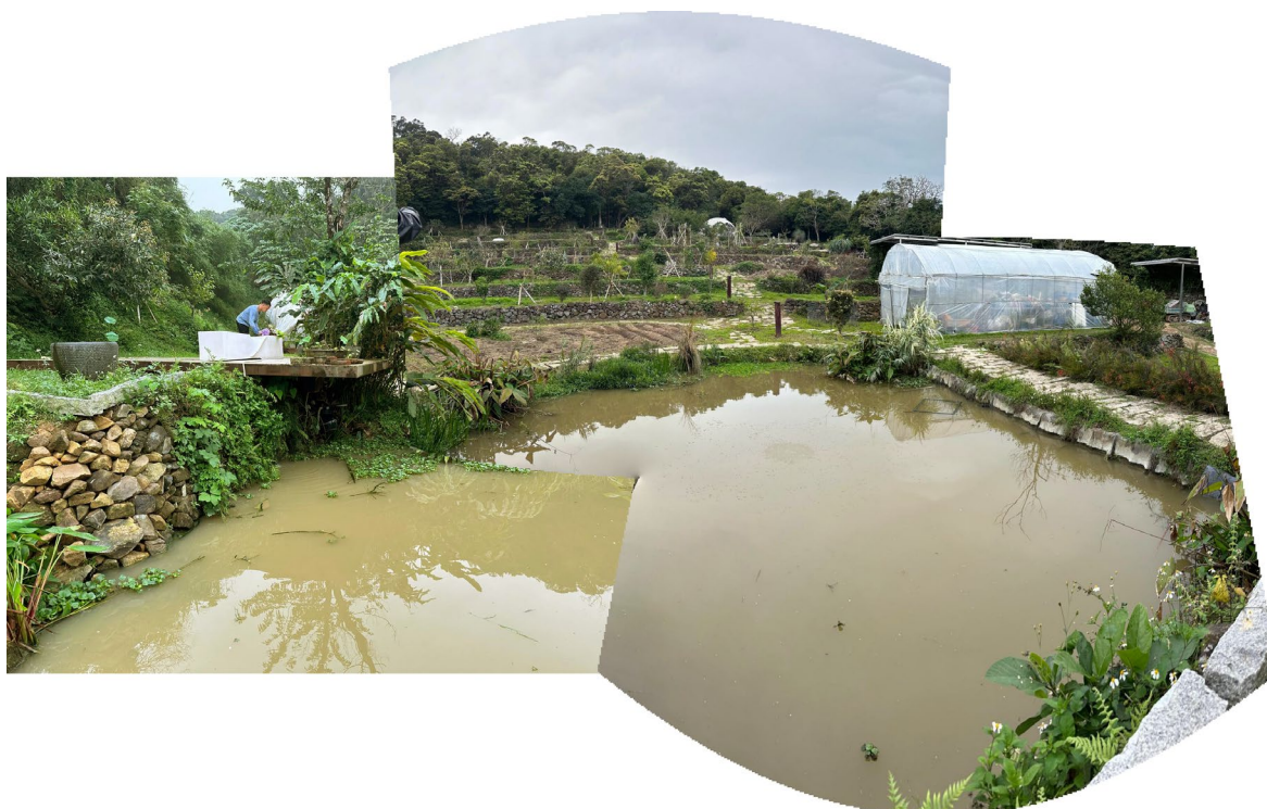
Figure 4.2 Existing Condition of the Lower Pond
