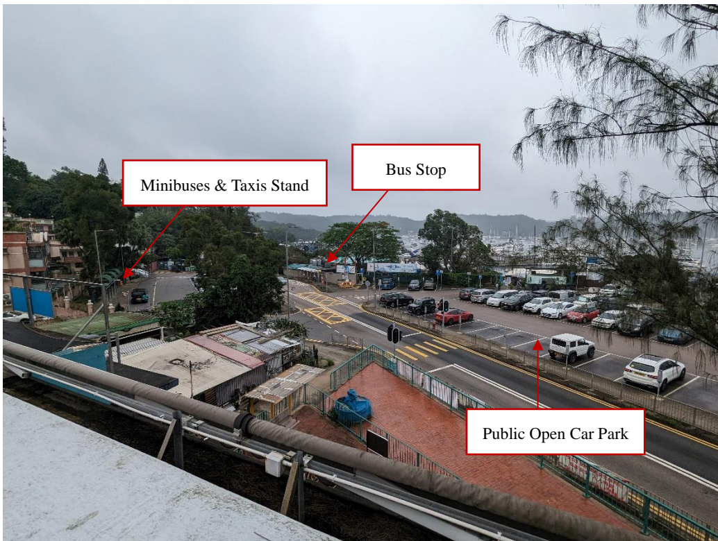
14. View from Roof & Transportation Facilities nearby
