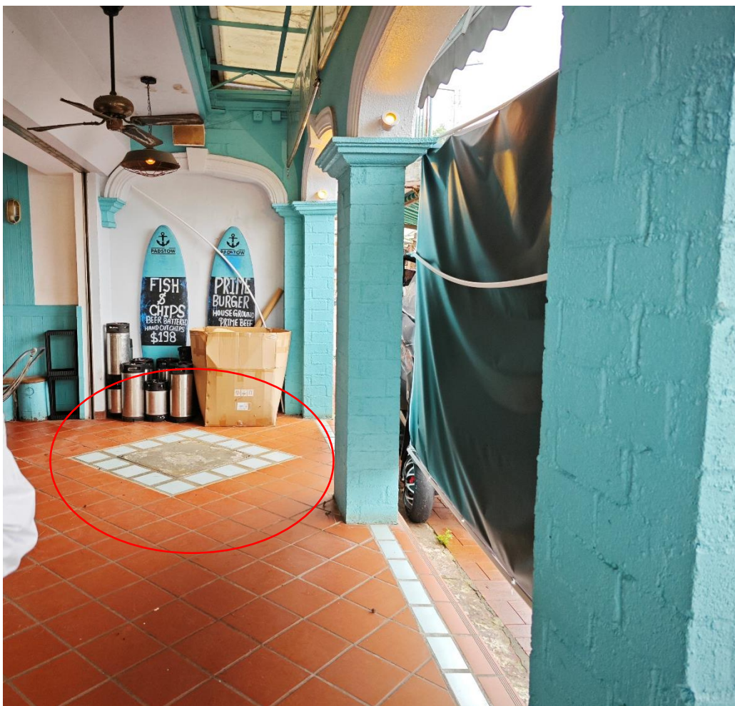
04. Foul Water Tank (E)
