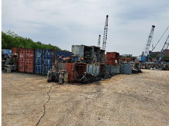
Photo 11: Construction Material Storage
