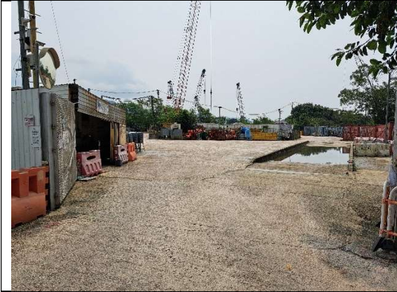
Photo 13: Open Area, Construction Storage Area and Car Wheels Washing Pool
