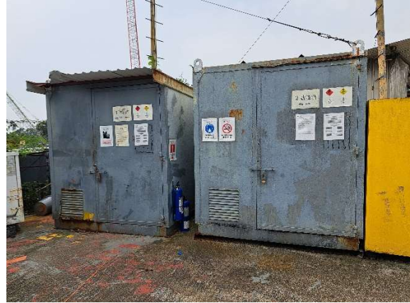
Photo 12: Chemical Storage Area
