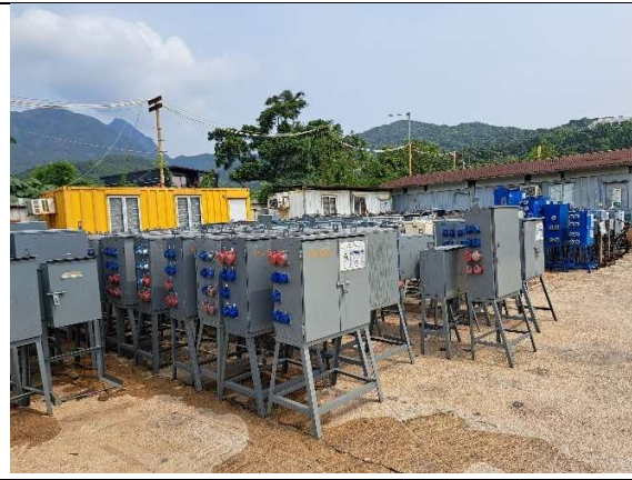
Photo 2: Construction Material Storage
