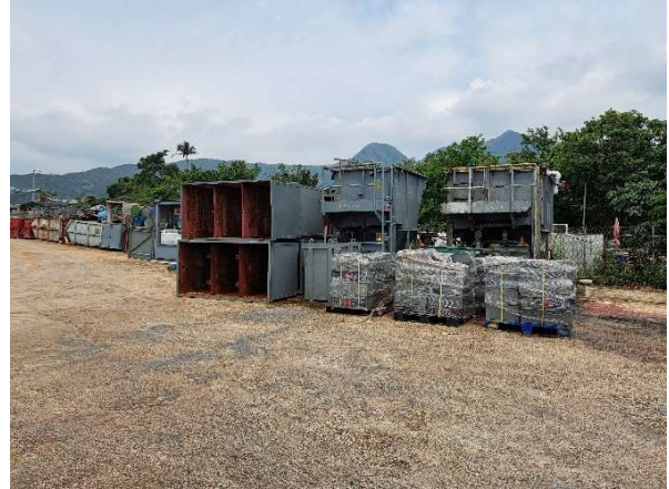
Photo 10: Construction Material Storage
