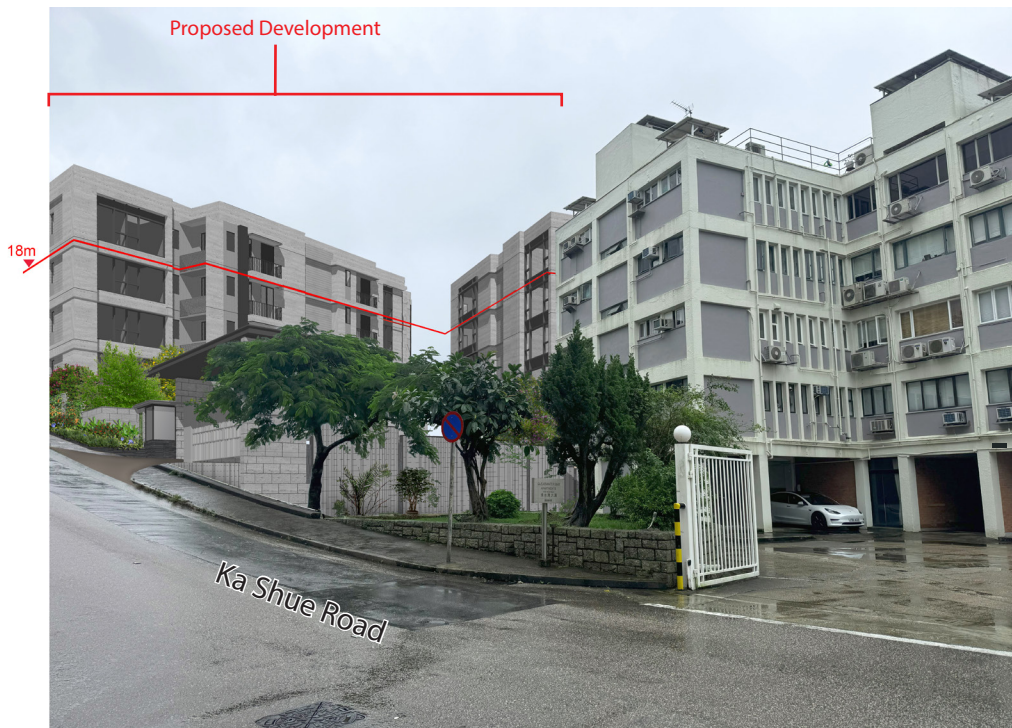
Photo B2 - Proposed Development at the Subject Site
