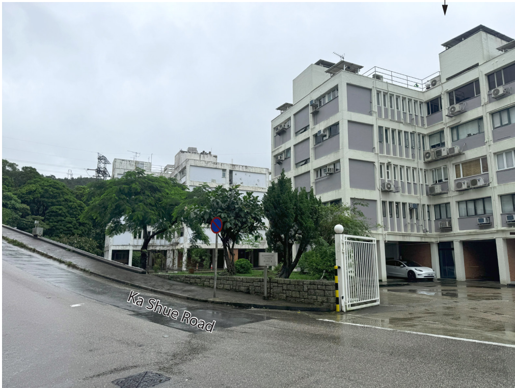
Photo B1 - Existing Conditions of the Subject Site
