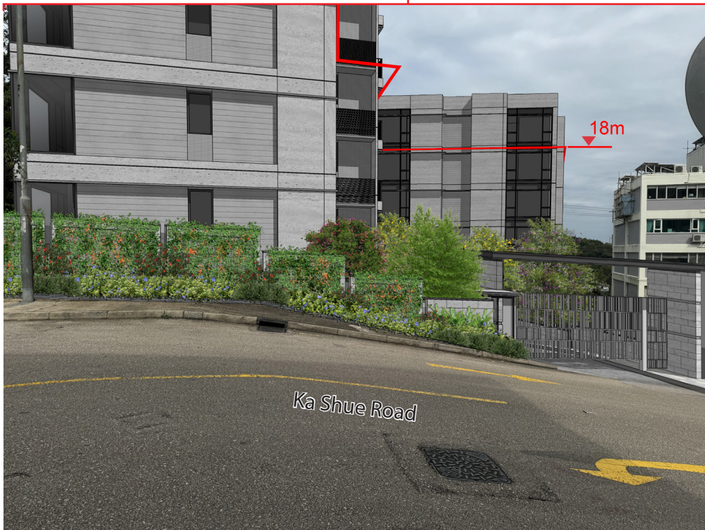
Photo E2 - Proposed Development at the Subject Site
