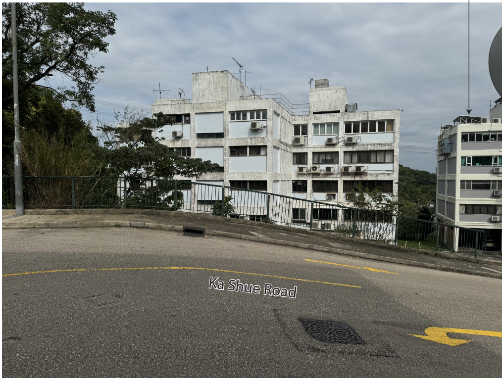
Photo E1 - Existing Conditions of the Subject Site
