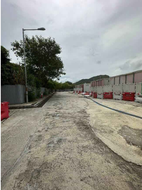
Inside of Project Site and fenced around the perimeter; MiC units, paved road and drains observed; potential contamination is anticipated as no stains and/or underground/above-ground storage tanks observed.
