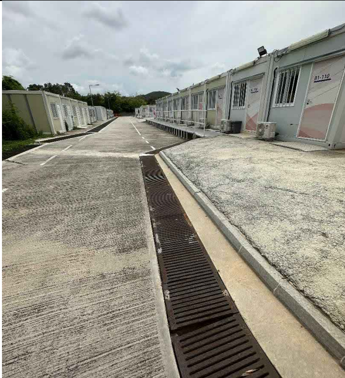
Within the San Tin CIF are paved roads and MIC units with A/C, drainages observed. No stains and/or underground/above-ground storage tanks observed.
