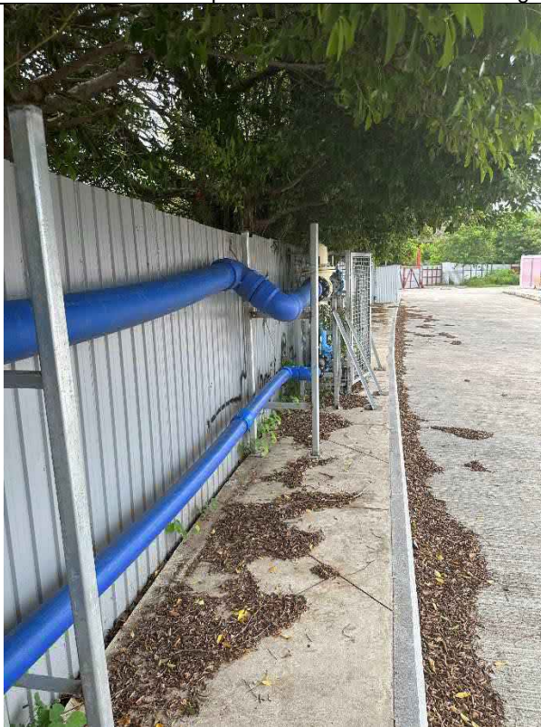
DSD pipes observed along fences around the perimeter.
