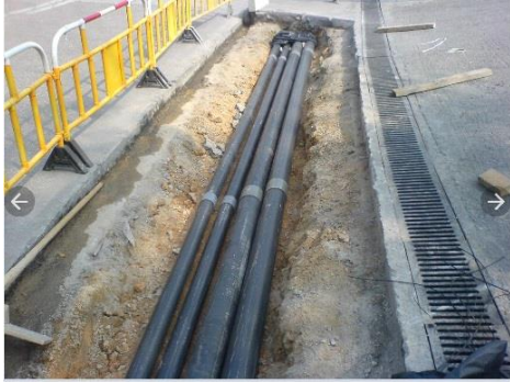
(3) Laying of Spare PVC Duck
