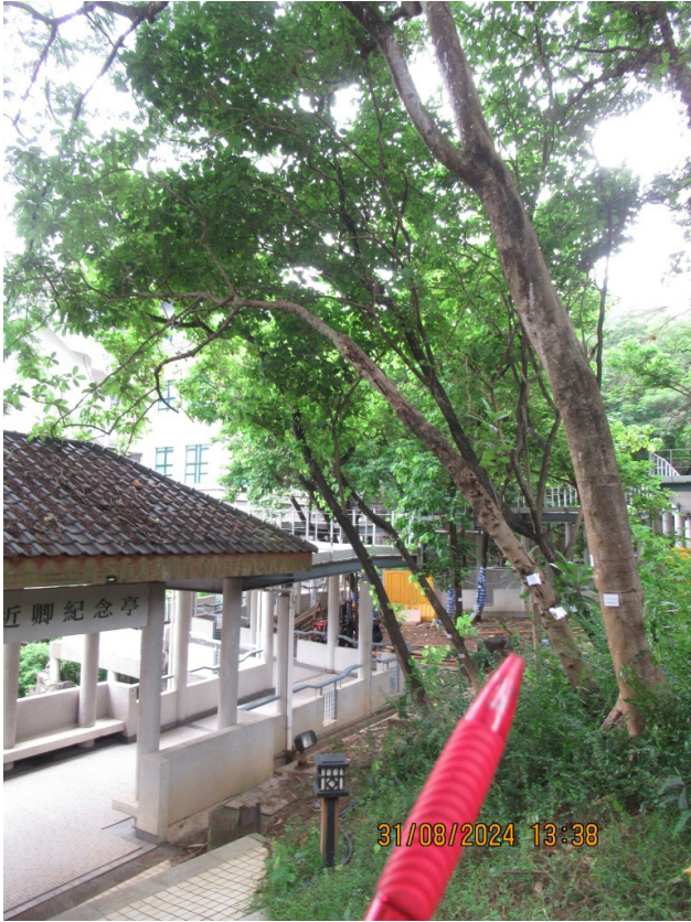
NS062 (OVERALL VIEW)
