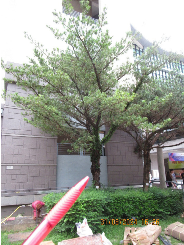
NS079 (OVERALL VIEW)
