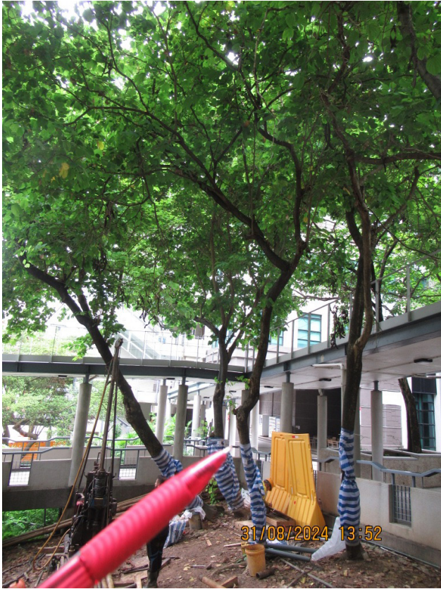
NS070 (OVERALL VIEW)
