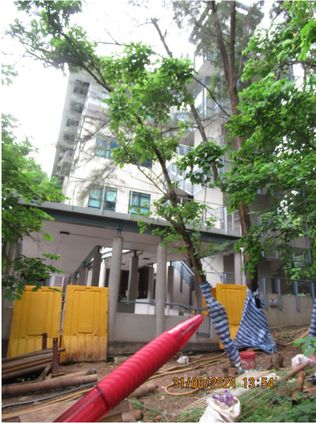
NS072 (OVERALL VIEW)
