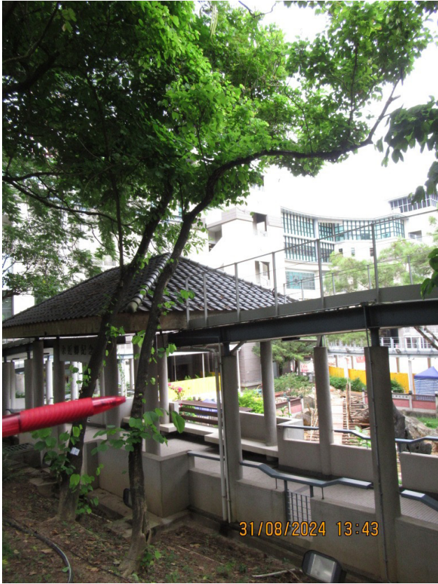
NS067 (OVERALL VIEW)
