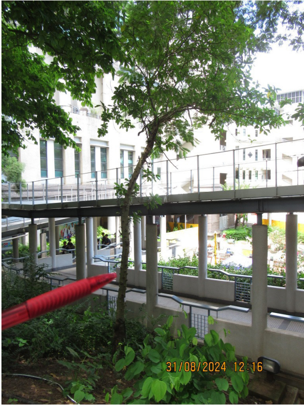
NS097 (OVERALL VIEW)
