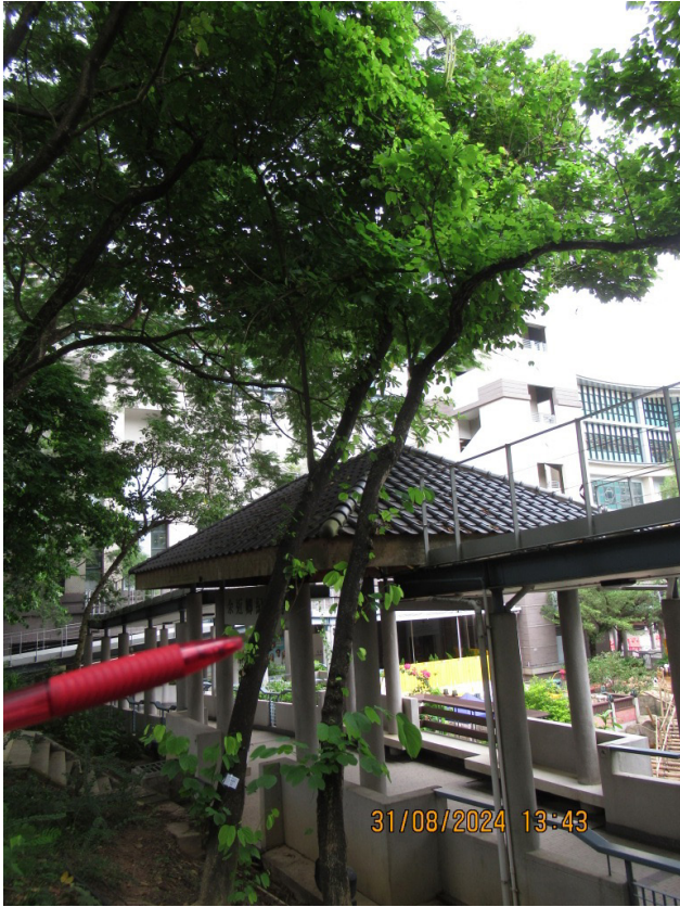
NS066 (OVERALL VIEW)
