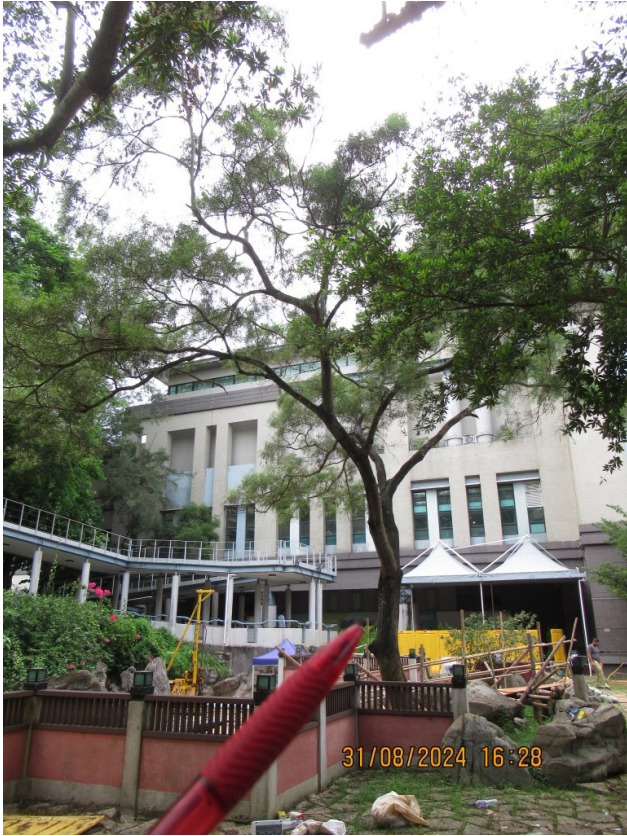
NS080 (OVERALL VIEW)
