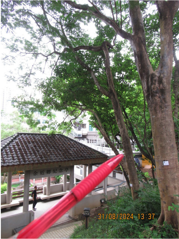
NS061 (OVERALL VIEW)
