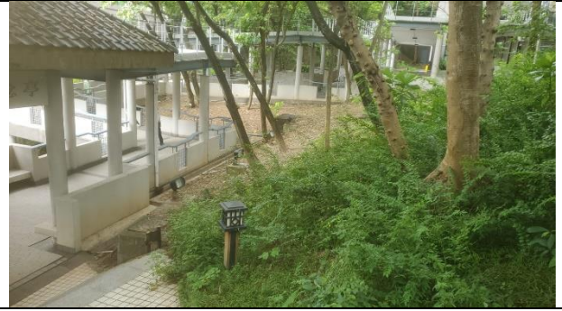
Photo 10: Slope at southeast
