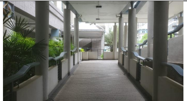
Photo 6: Concrete Bridge at Northeast
