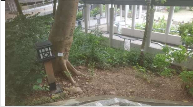
Photo 9: Slope at Southwest
