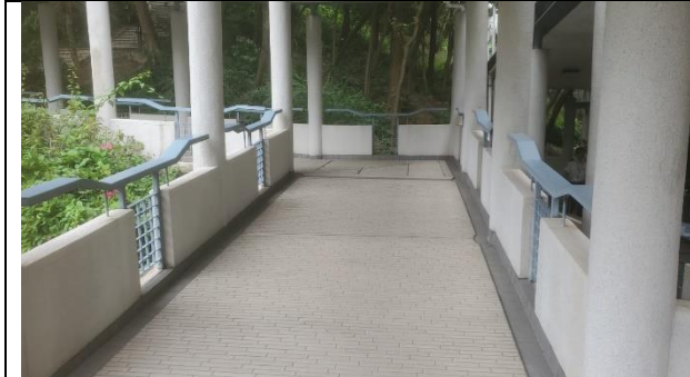
Photo 7: Concrete Bridge at Northwest
