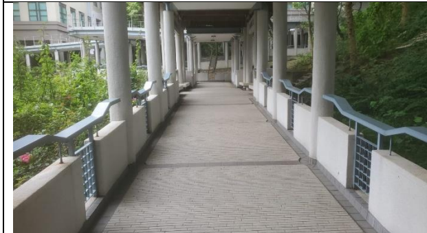
Photo 5: Concrete Bridge at Middle
