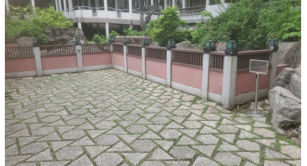
Photo 4: Northwest portion of the Application Site
