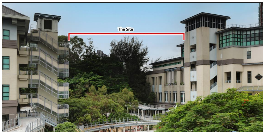
Photo 2.1: The Site viewed from the North
