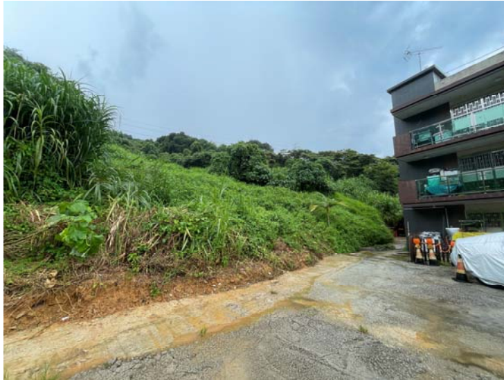
Plate 4: Viewing the toe of the Existing Slope and Application Site
