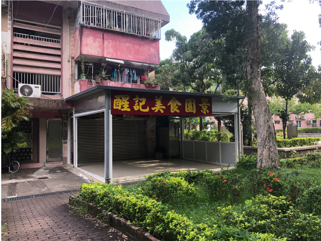
Photo 7: Design of the built-over structure previously that was under refurbishment
