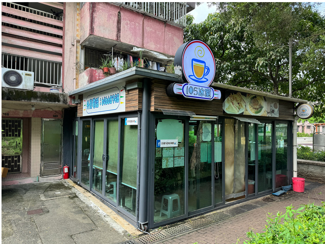
Photo 8: Current design of the built-over structure
