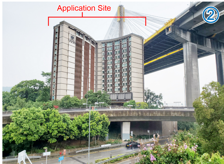
The Application Site is currently occupied by an existing hotel named Royal View Hotel
