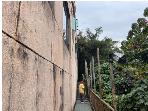
Photo 6: South of the site.
