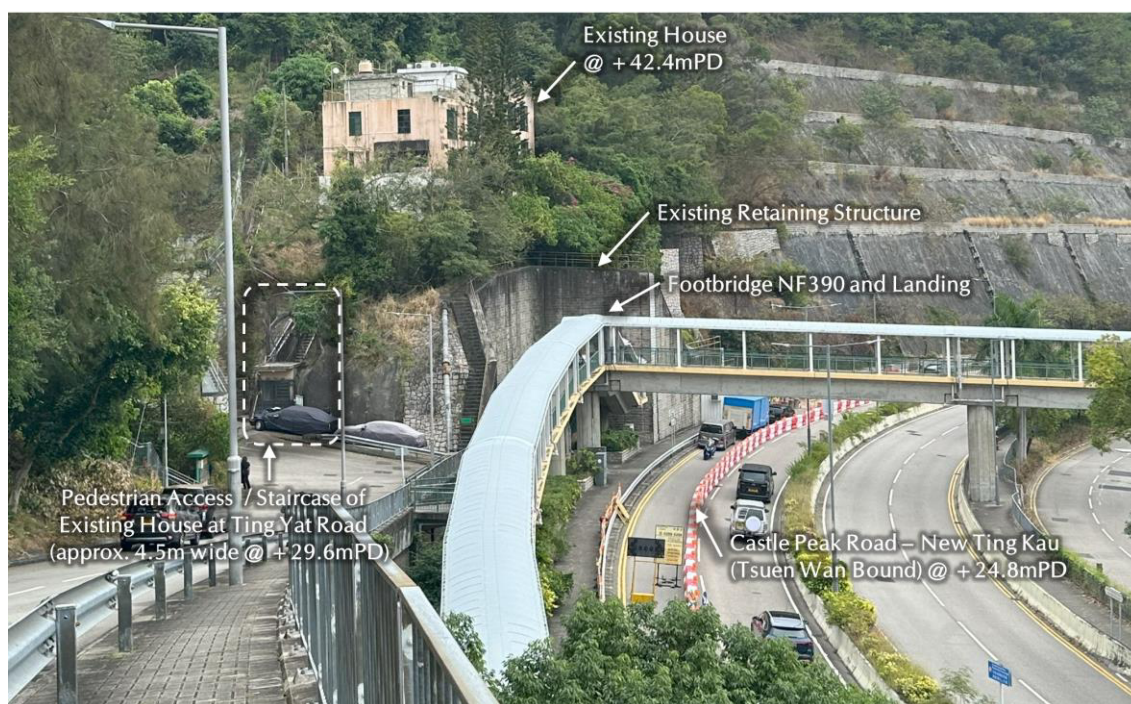
Photo 2.1 – Existing Condition of the Subject Site
