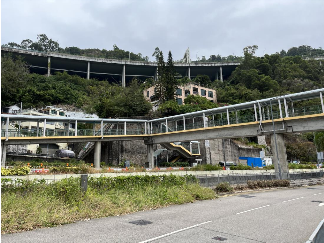
General view at left portion of development site (Facing west)
