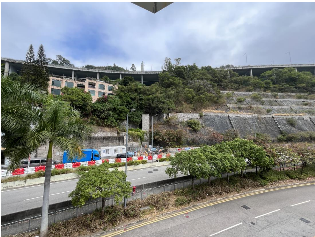
General view at right portion of the development site (Facing west)
