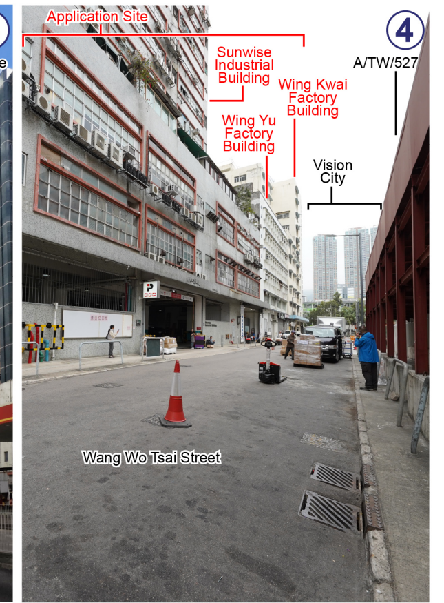
The existing industrial buildings at the Application Site viewing from Wang Wo Tsai Street
