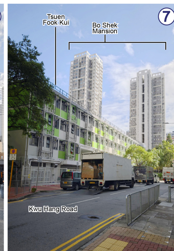
The Transitional Housing "Tsuen Fook Kui" and HOS "Bo Shek Mansion"
