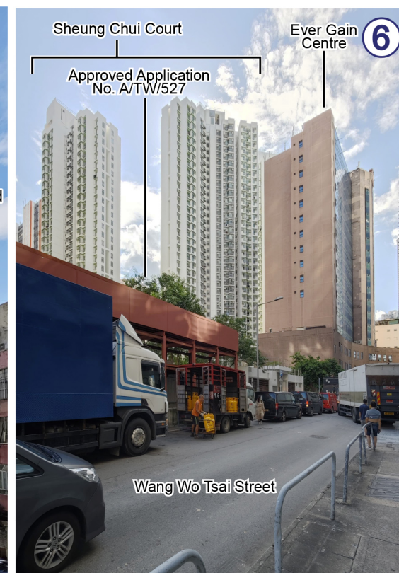
The existing industrial development and HOS "Sheung Chui Court" at Wang Wo Tsai Street
