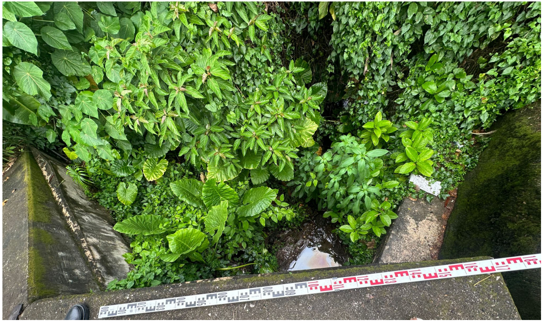
Photo of Existing Box Culvert
