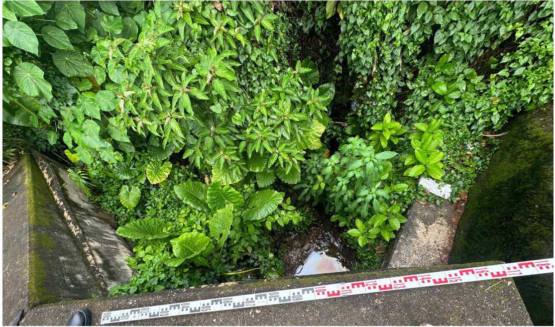
Photo of Existing Box Culvert
