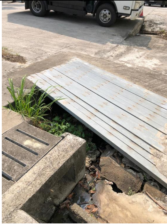
View 2a Existing 600UC and 500UC its connection point by catchpit
