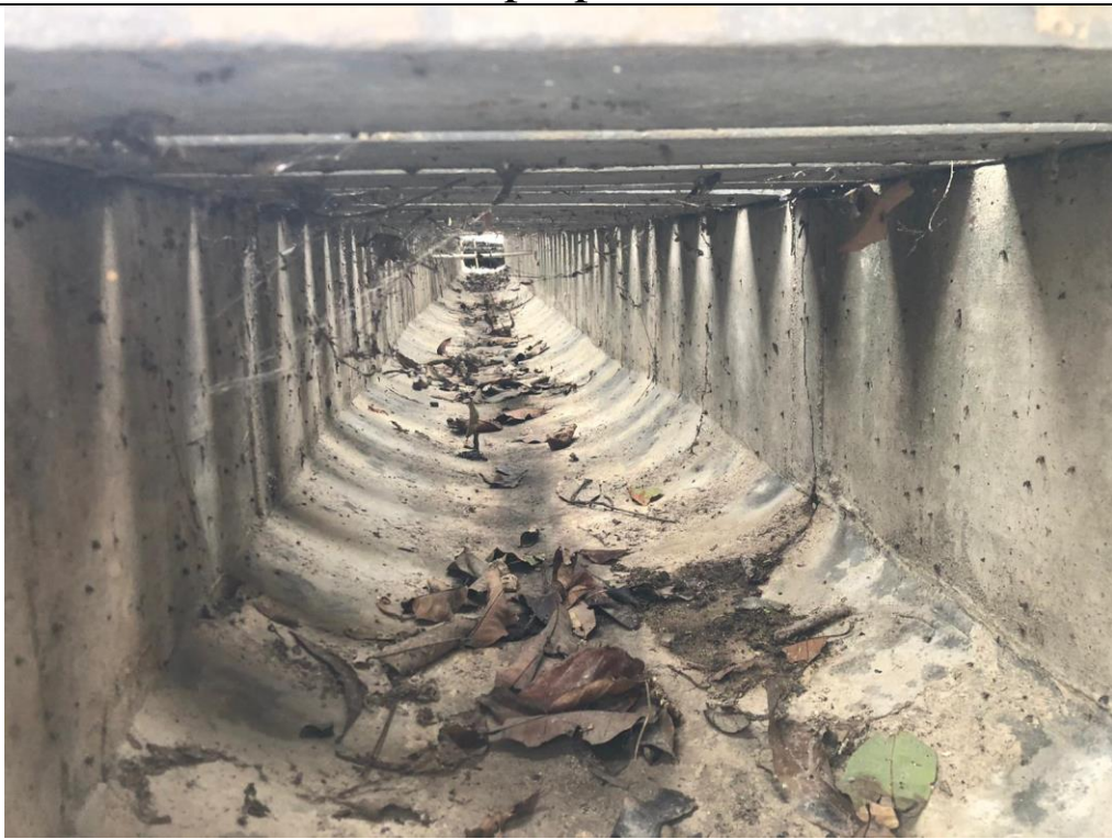
View 3c Internal Condition of Existing 500UC besides proposed site
