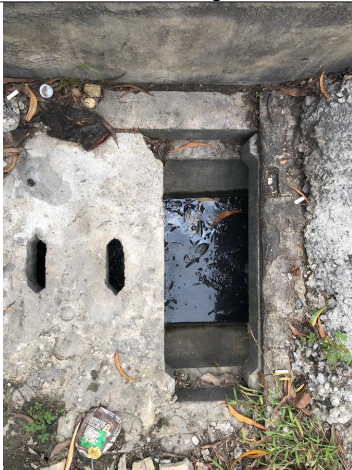
View 1b Internal Condition of Existing 600UC
