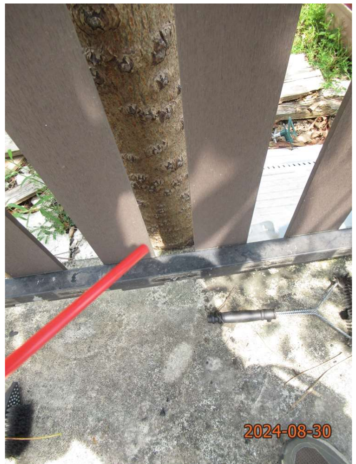
T5 Tree base embedded to concrete structure
