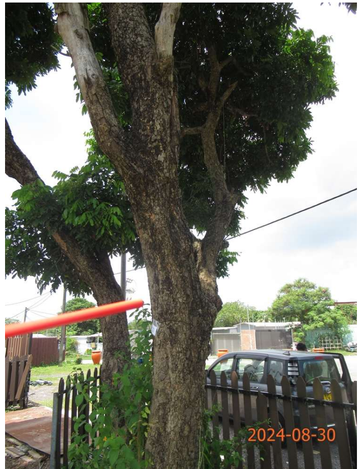
T2 (Trunk condition)
