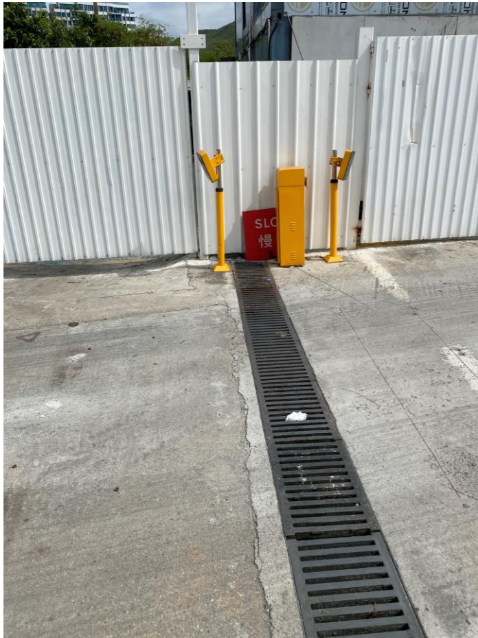
Photo 1: U-Channel at Entrance of Project Site (Site 1)
