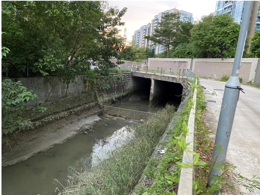
Photo 1: Box Culvert north of the Project Site
