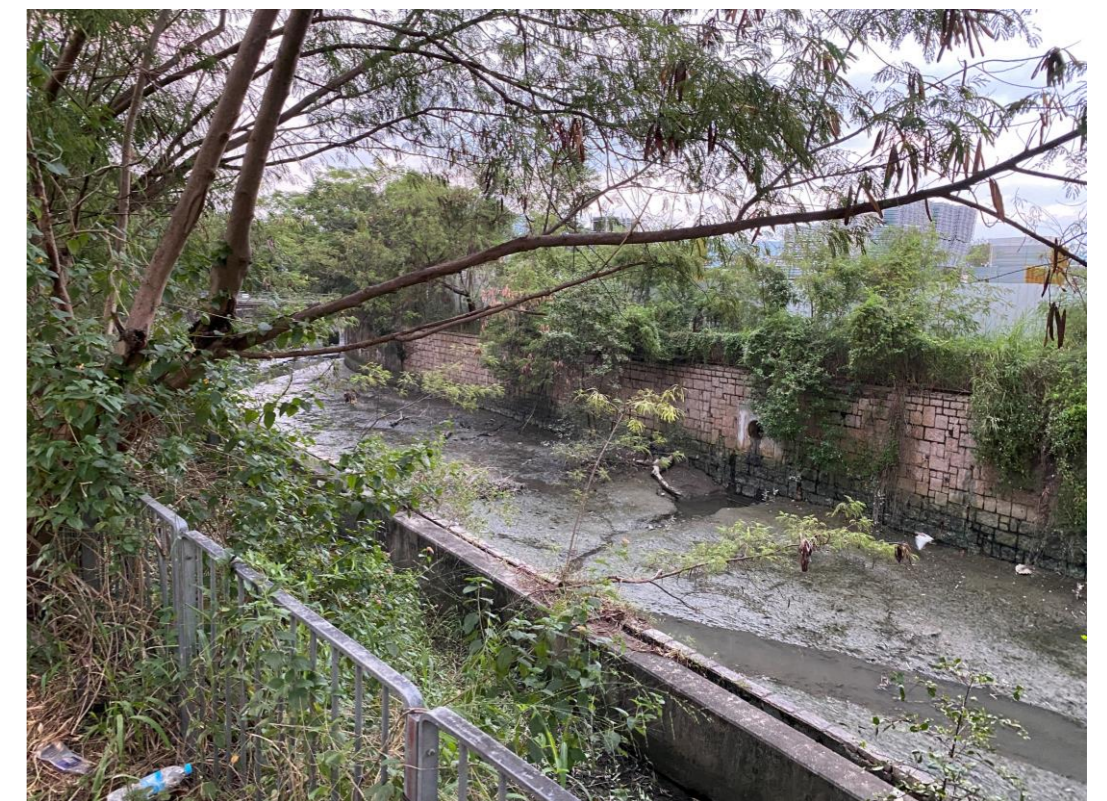
Photo 2: Box Culvert north of the Project Site
