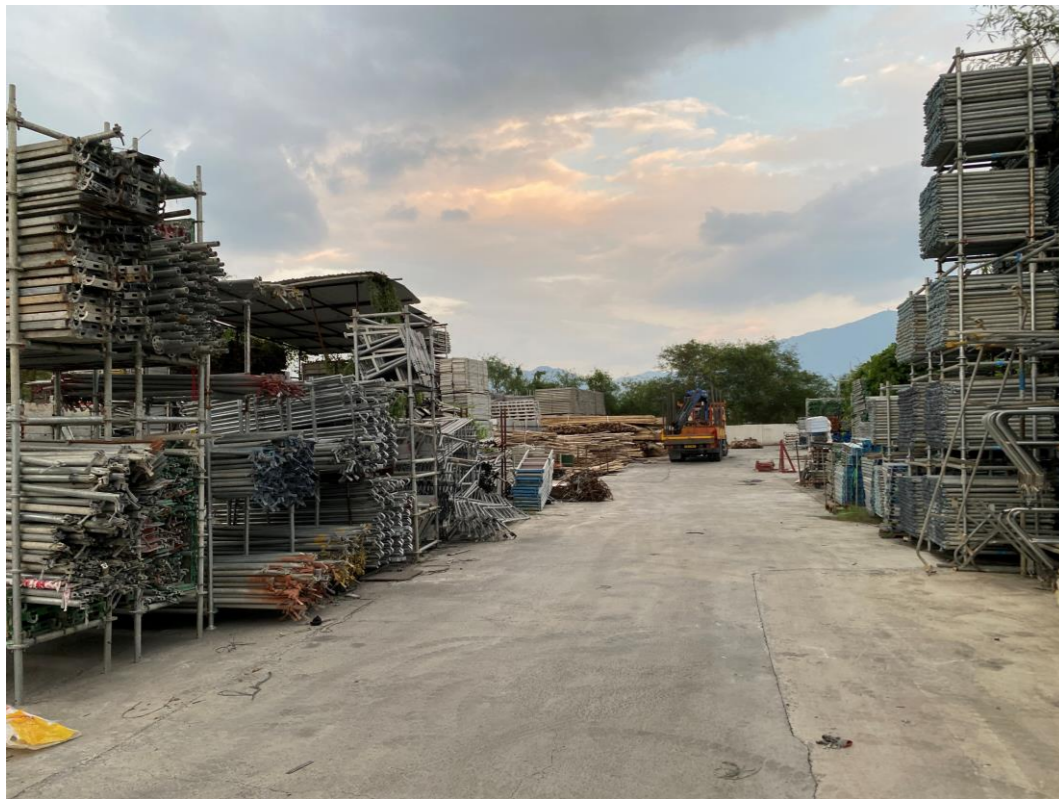
Photo 3: No U-Channel at Site 2 of Project Site
