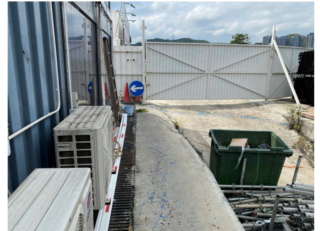
Photo 2: U-Channel at Entrance of Project Site leading north in Site 1
