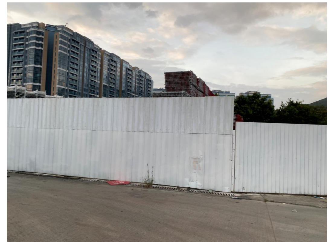
Photo 2: Hoarding without Concrete Footing
