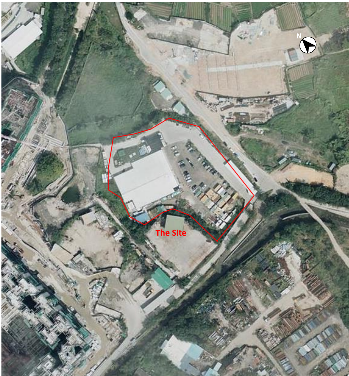
Figure D - 6 Aerial Photograph in Year 2015
