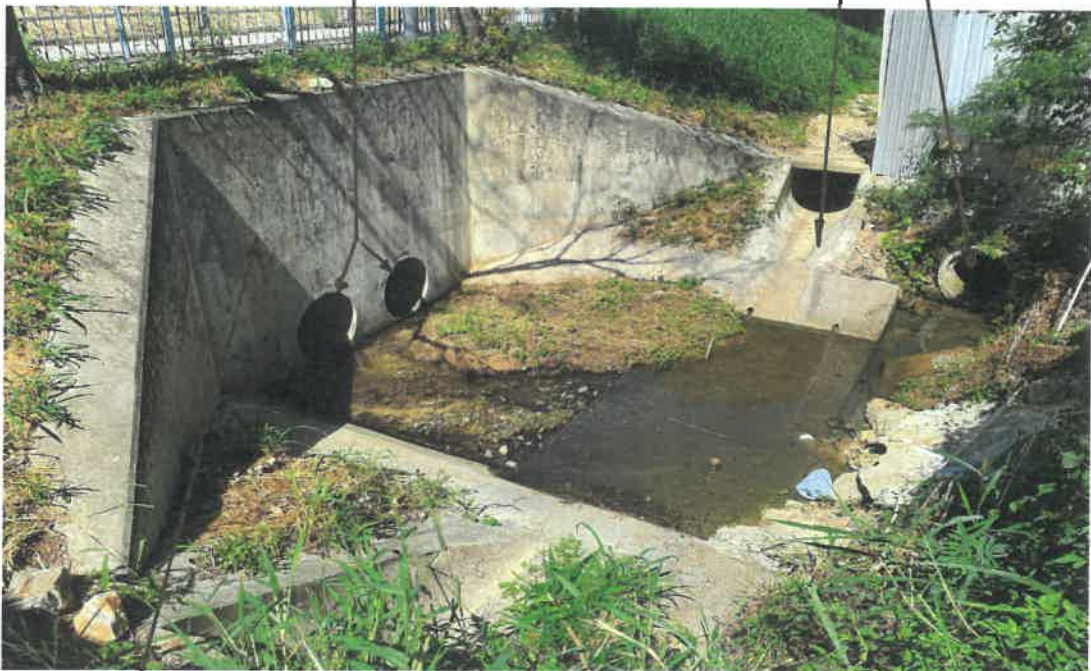
Existing Public Inlet Structure
