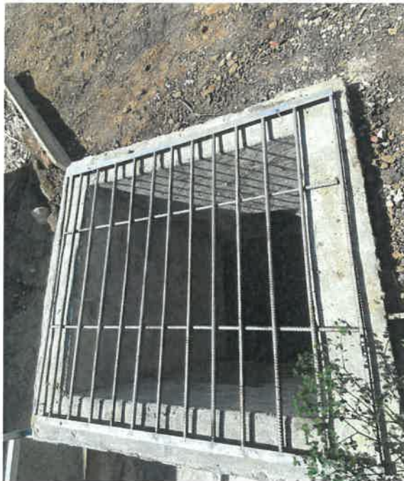
PHOTO NO. 6 Existing Catchpit C1 with 600mm Underground Pipe Discharging Water to Existing Public Inlet Structure
