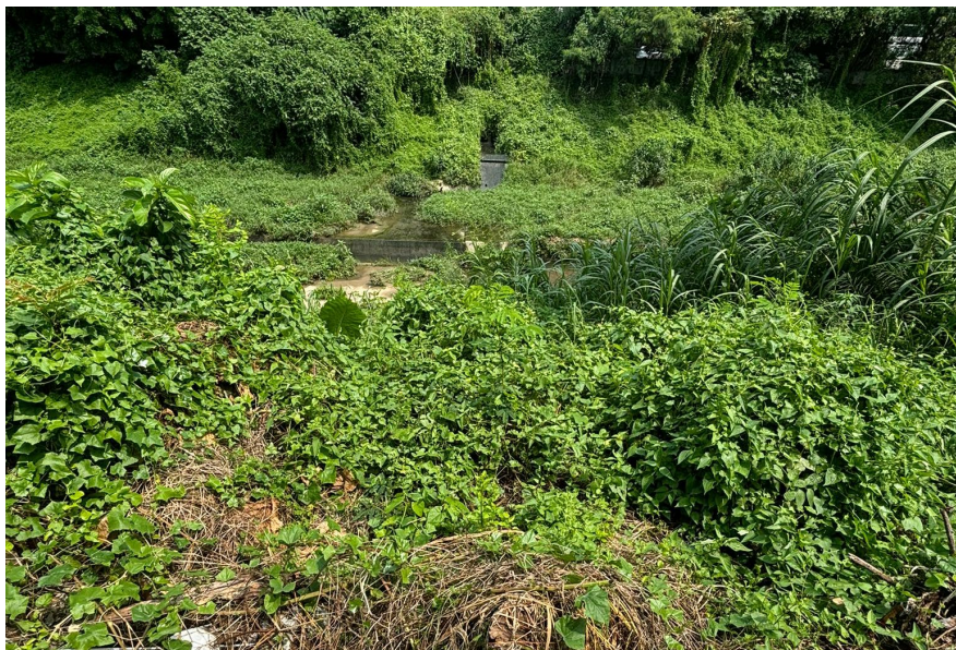
Drainage pipe underneath connects to the outfall at Kam Tin River
