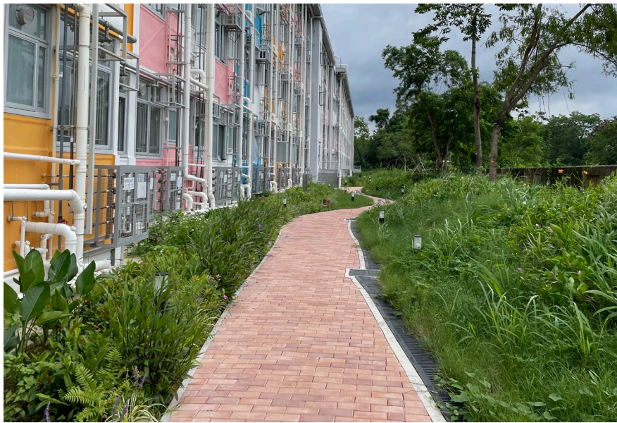
U-channel next to the landscaping
