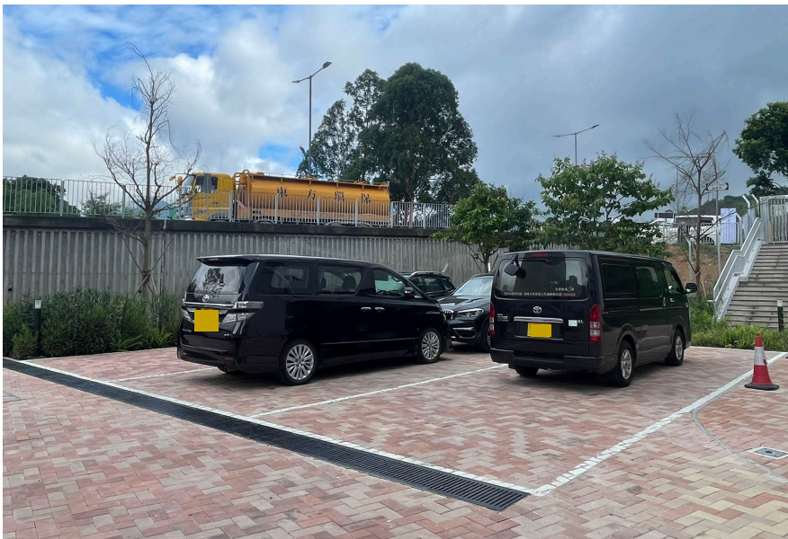
U-channel next to car parking
