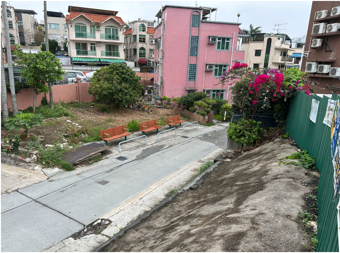
VIEW C Adjacent Area of the site
