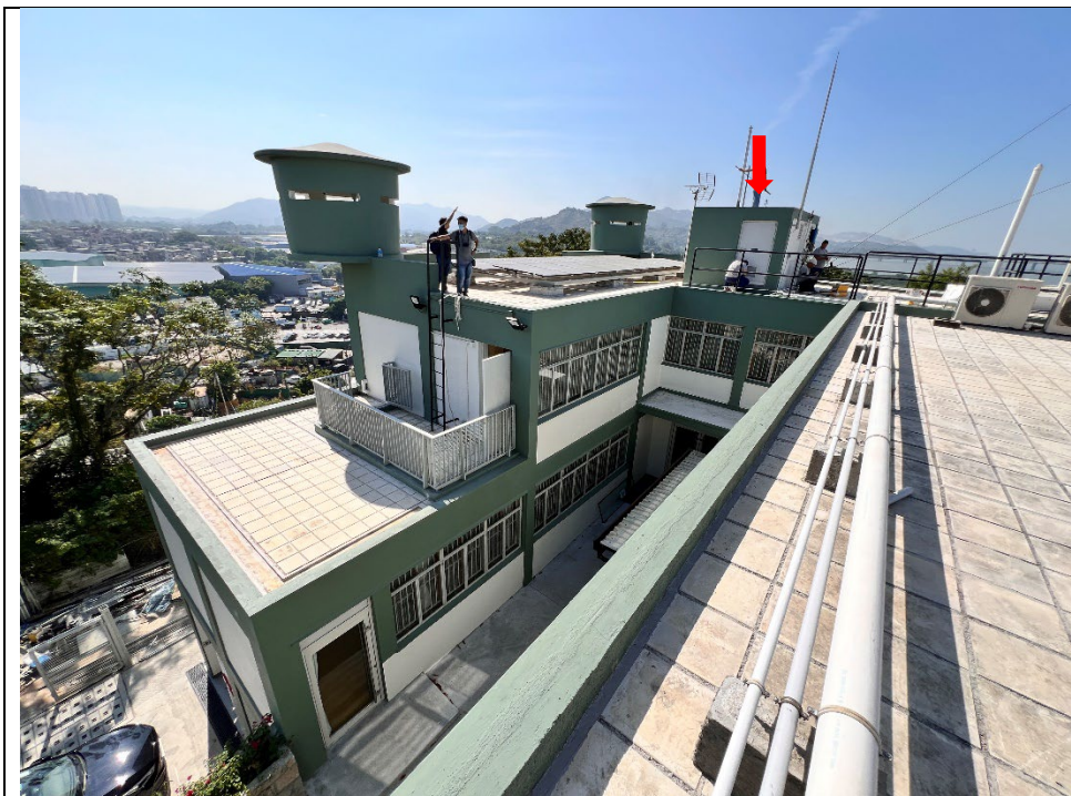
Photo 2. The Subject Site (red arrow) on top of a flushing/cleansing tank & pumps room on the rooftop of Former Lau Fau Shan Police Station
