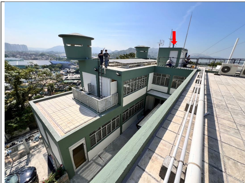
Photo 2. The Subject Site (red arrow) on top of a flushing/cleansing tank & pumps room on the rooftop of Former Lau Fau Shan Police Station
