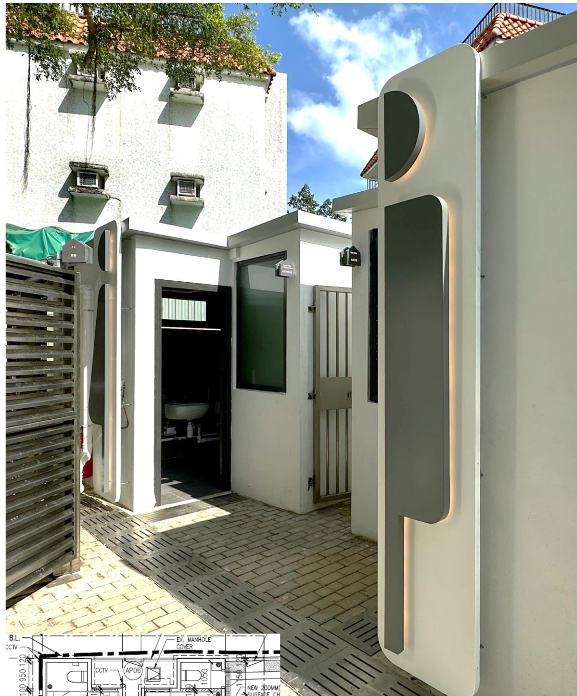
V1 LAVATORY ENTRANCE
