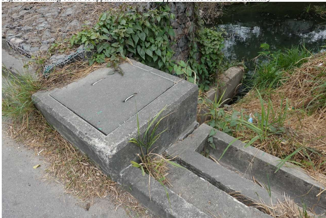
Figure 2. Existing outlet of application site
