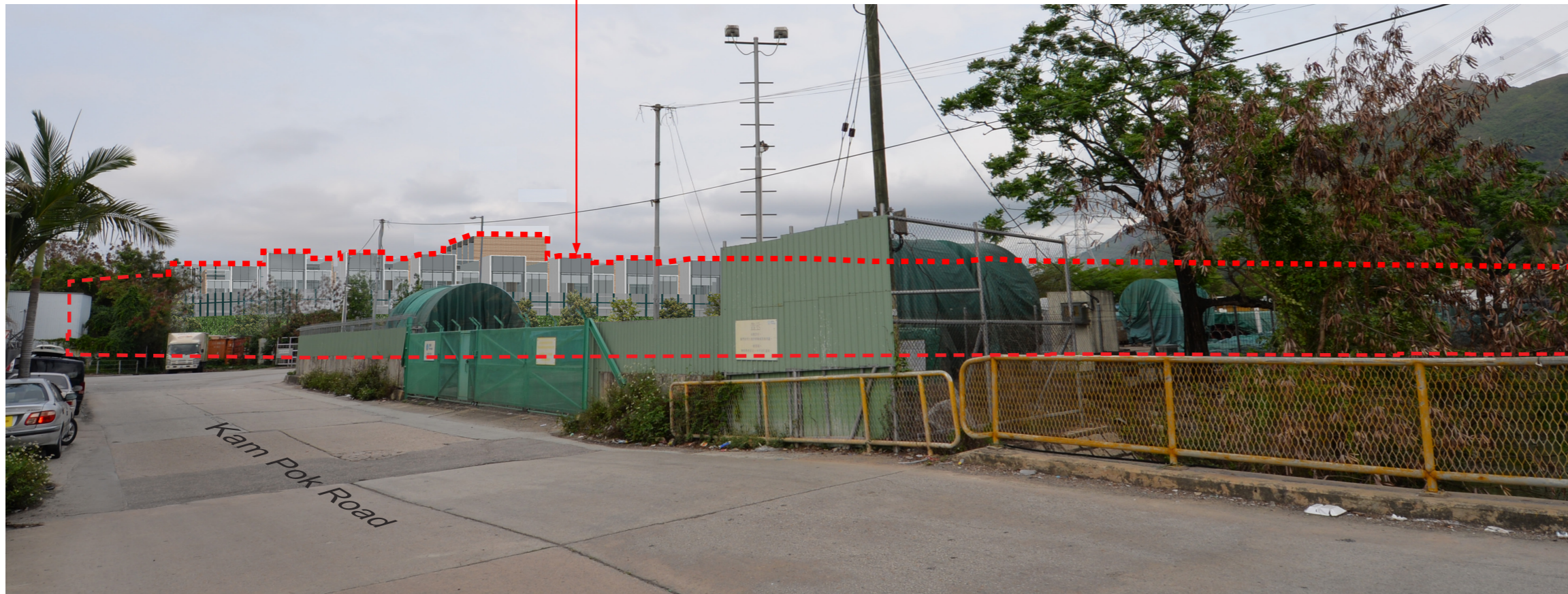
VP4: View looking towards the Subject Site from Kam Pok Road (with Proposed Scheme)
