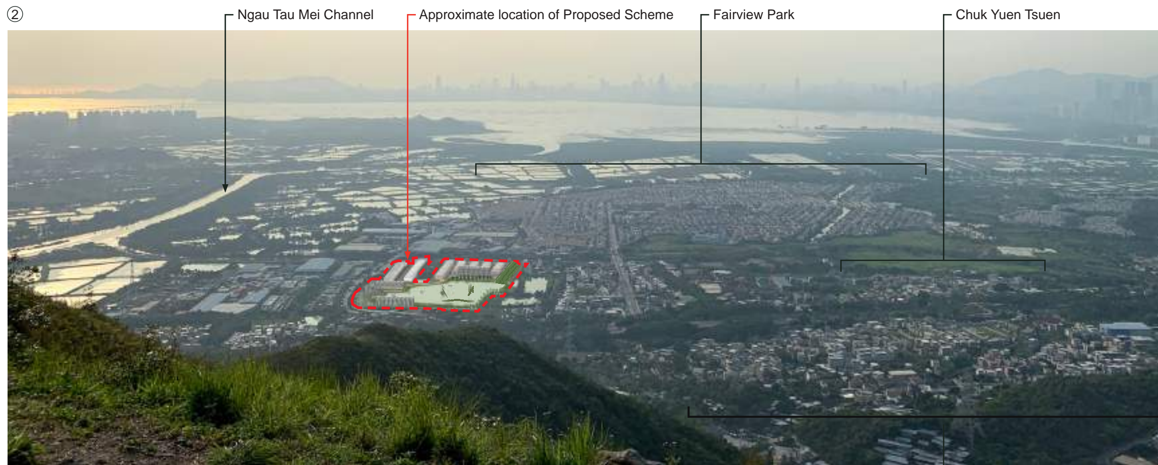
VP11: View looking towards the Subject Site from Kai Kung Leng (with Proposed Scheme)
