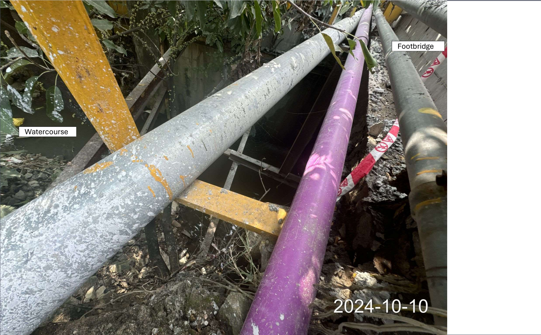
Figure 3-7: Photo of the Existing Watercourse underneath Footbridge
