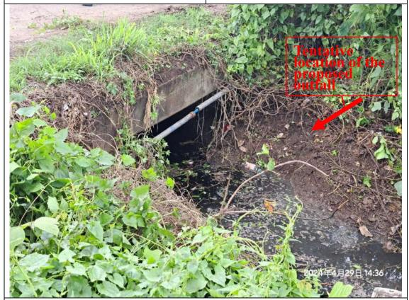
**Plate 8** – Existing watercourse to the south receiving stormwater discharge from the subject site and discharging into the existing branch channel of the Kam Tin Main Stormwater Channel
