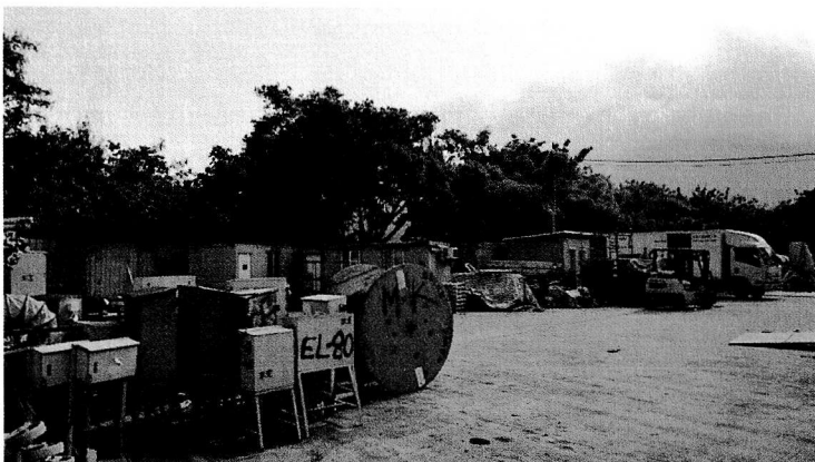
Photo No. 6 To the north of the proposed site area. It will be covered with metal shelters for warehouse.
