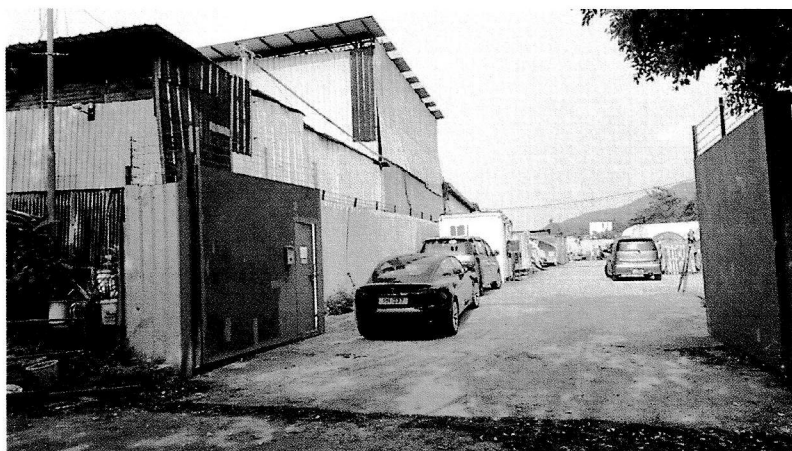
Photo no.3 A general view of the site entrance with a 12.0-meter gate opening.
