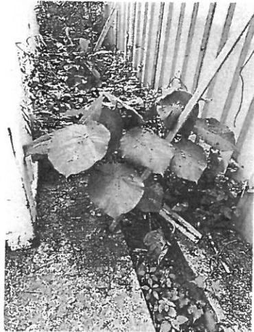
Photo No. 5 At the north bound and east bound of the proposed warehouse site is an existing 300mm U-channel running along.
