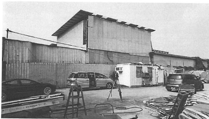
Photo No. 2 Viewing to the south side, along the boundary is the metal fence. Beyond is sheltered temporary warehouses with ground level at +20.50mPD to +20.01 mPD.
