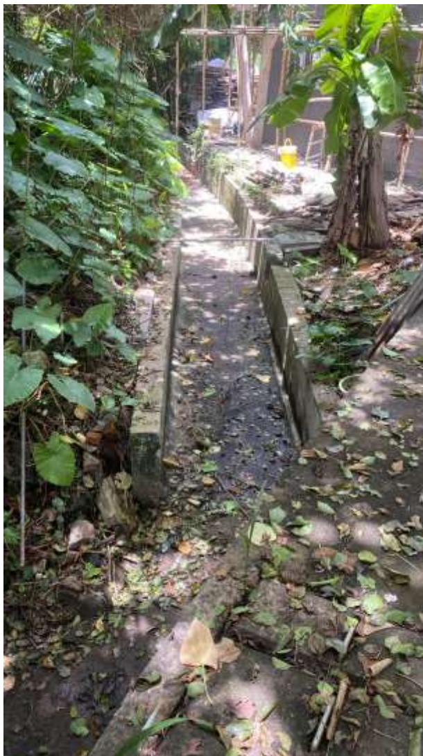
Photo showing the existing drainage facilities
