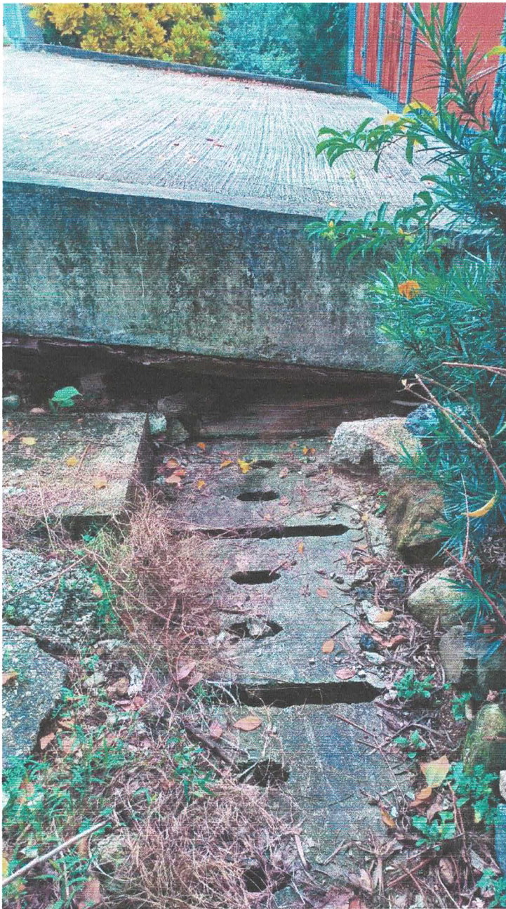
Photo 3 – Run-in Constructed under A/YL-SK/306 and U-Channel below
