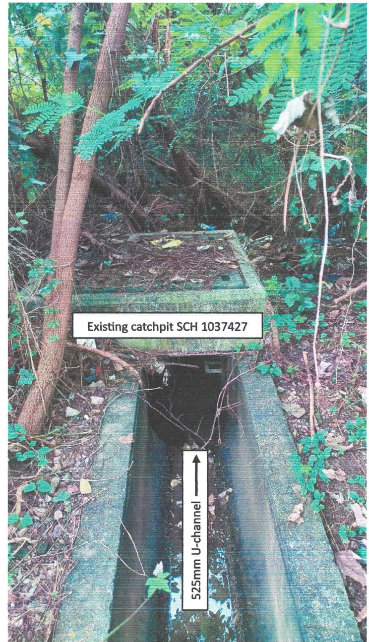
Photo 4 – Existing Catchpit and U-channel below Ko Sheung Road
