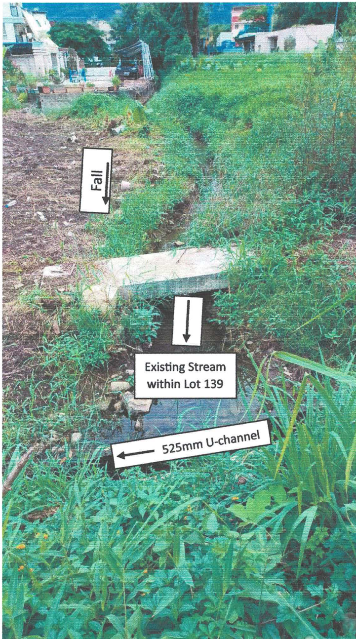
Photo 5 – Existing Stream within Lot 139
