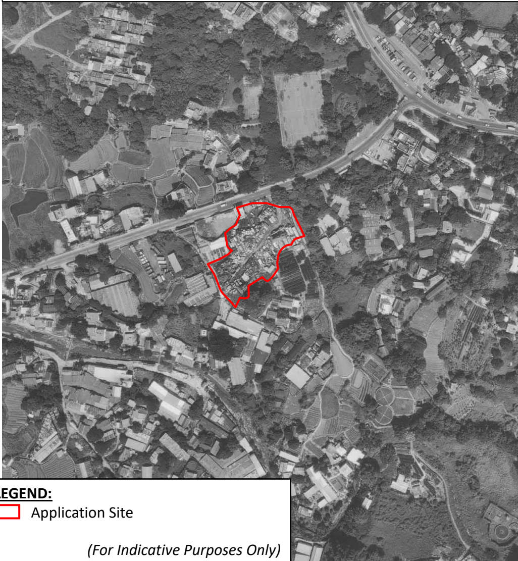
Extract of Aerial Photo No . A22942 dated 5.10.1995
