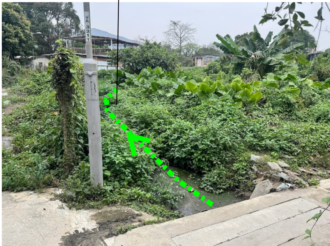
Existing Village Drain A
